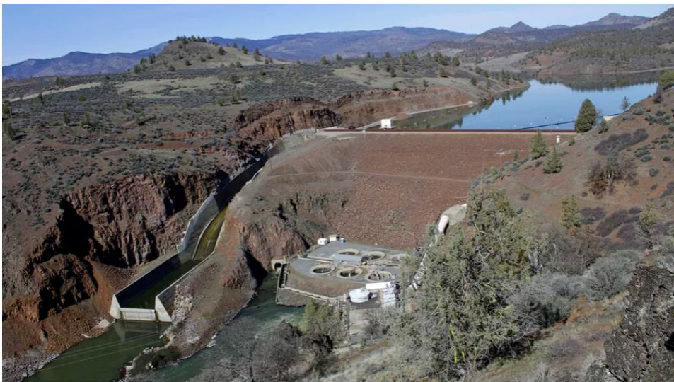
The Iron Gate Dam, powerhouse and spillway is seen in 2020 on the lower Klamath River near Hornbrook, Calif. Gillian Fleccus/AP
